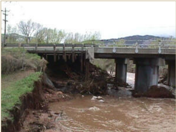
State Highway 24 at Fountain Creek
