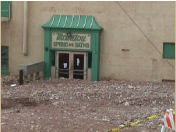
Debris Flow at the Manitou Spring and Bath House
