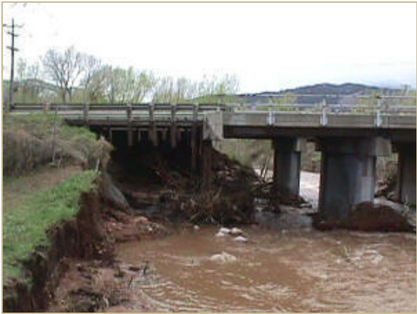
State Highway 24 at Fountain Creek
